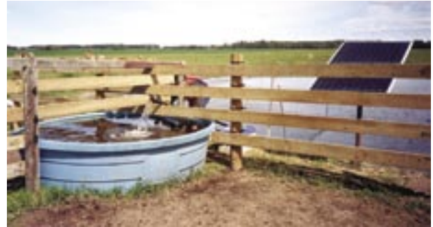
Solar systems provide another option when pumping water at a remote location
